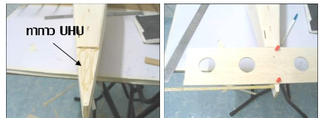
1. Center the stabilizer on the stab saddle
